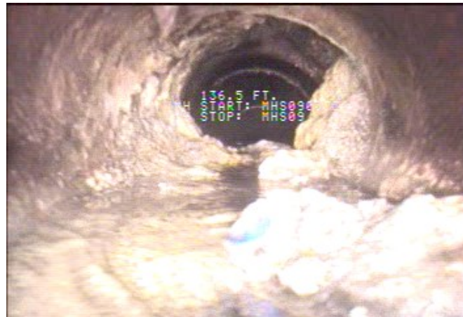
SEWER MAIN (LATERAL AT RIGHT OF EACH IMAGE)
